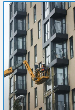
Cladding removal at Kennedy Gardens, Billingham
